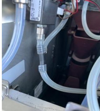
11. Disconnect the silicone hose from the bottom of the vacuum
