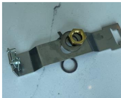
14. Transfer Fiber Gasket, Bracket, washer and nut to new boiler
